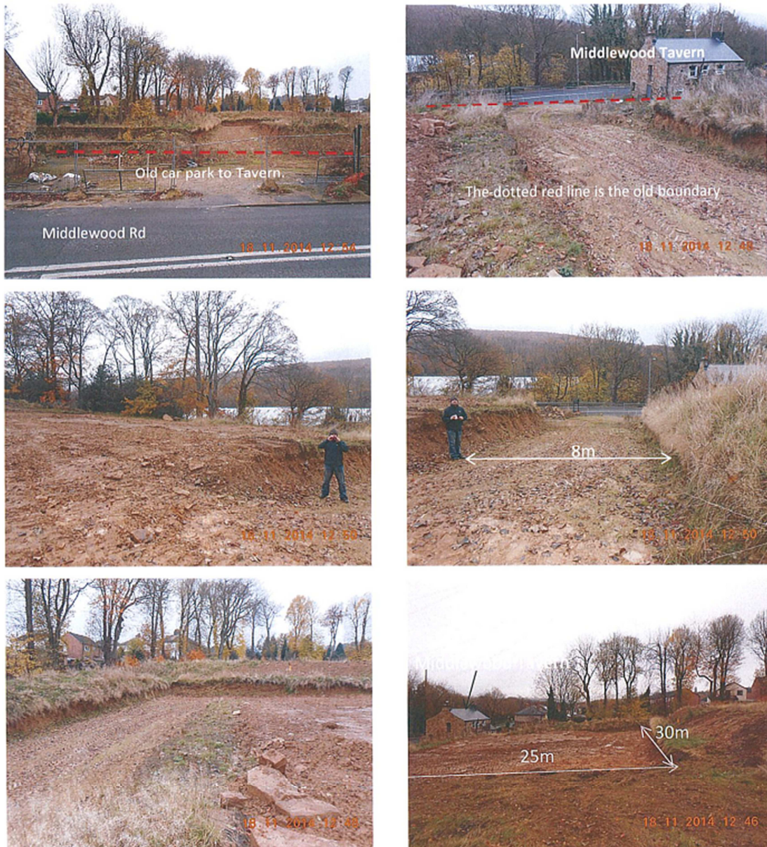
Photographs / Site Plan, Land off Middlewood Road North
